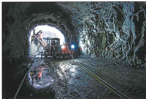
(a) Tunnelling work at the 370 MW Lysebotn upgrading project. Photo: Lyse.
