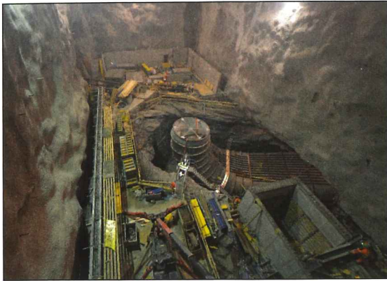
(b) New powerhouse extension at the Lower Røssåga powerplant. Photo: Statkraft.
